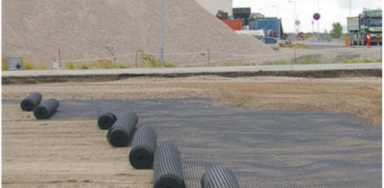
Representative pavement geogrid deployment over prepared formation.
