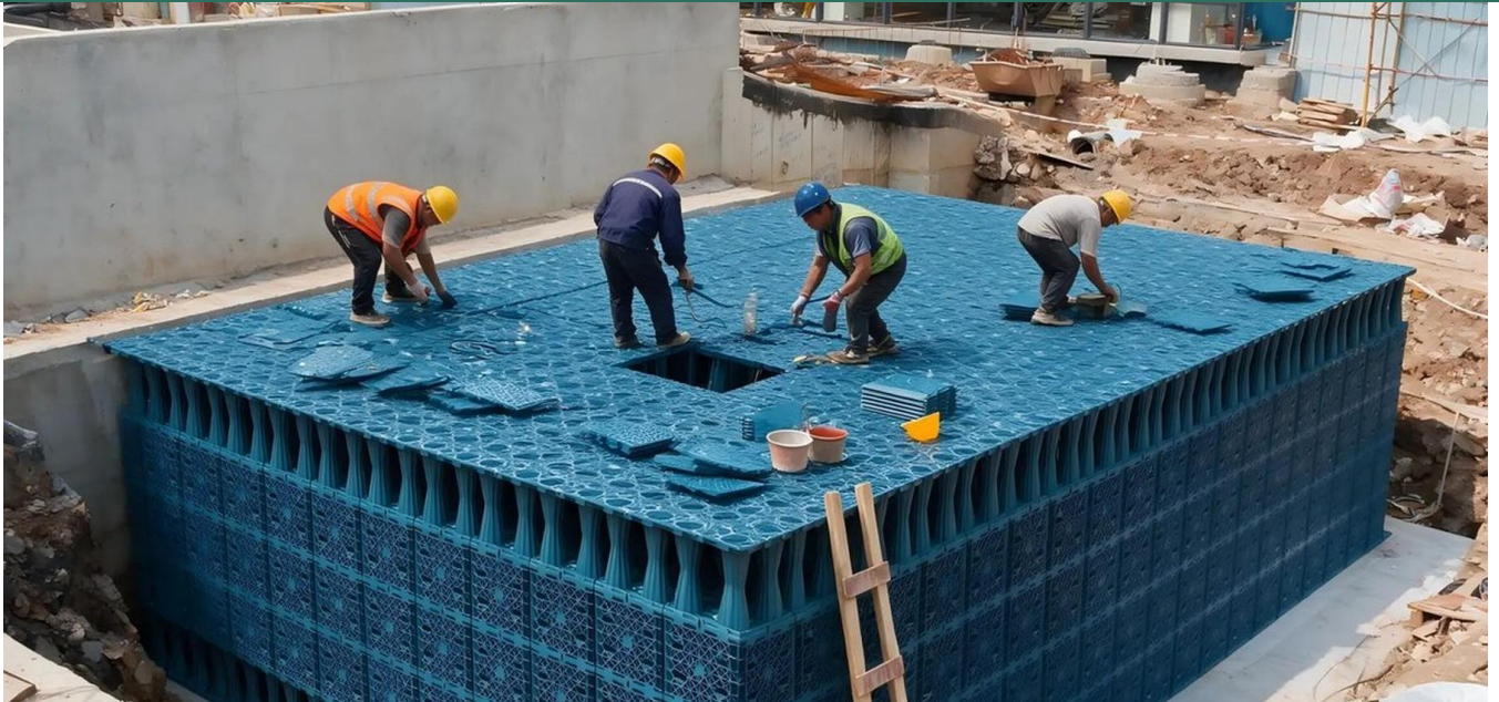
Representative M2025 modular tank assembly during installation.
