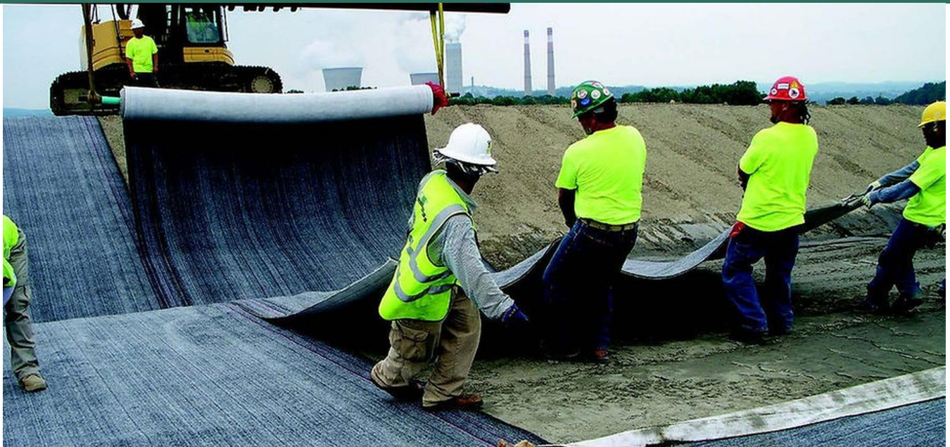
Representative GCL installation and overlap control.
