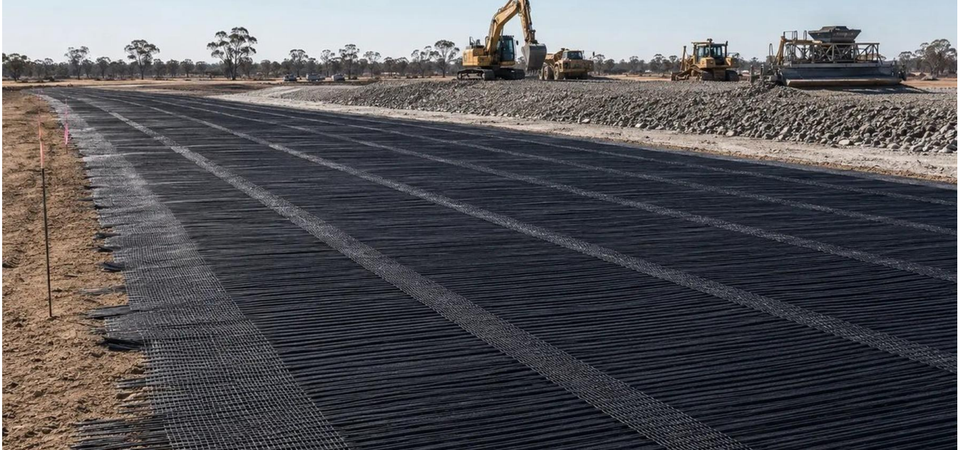
Representative basal reinforcement and aggregate-placement application.
