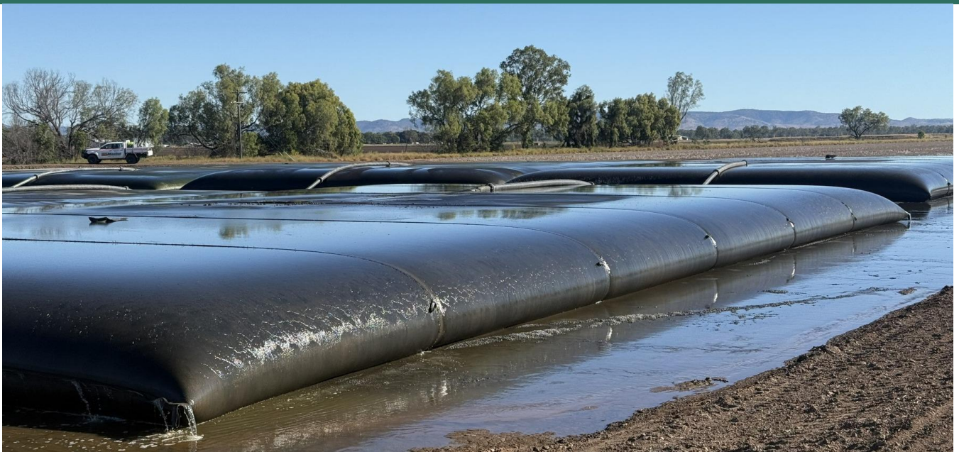
Representative large geotextile dewatering containers operating on a lined pad.
