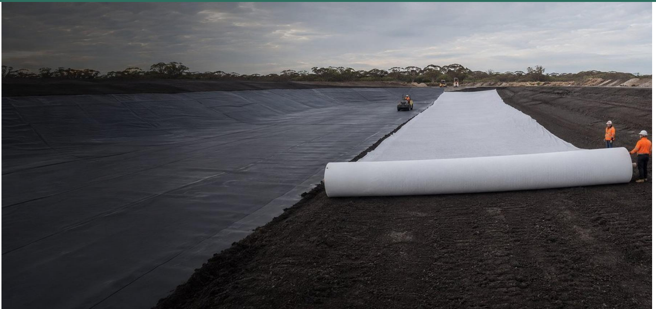
Representative nonwoven installation within a containment system.
