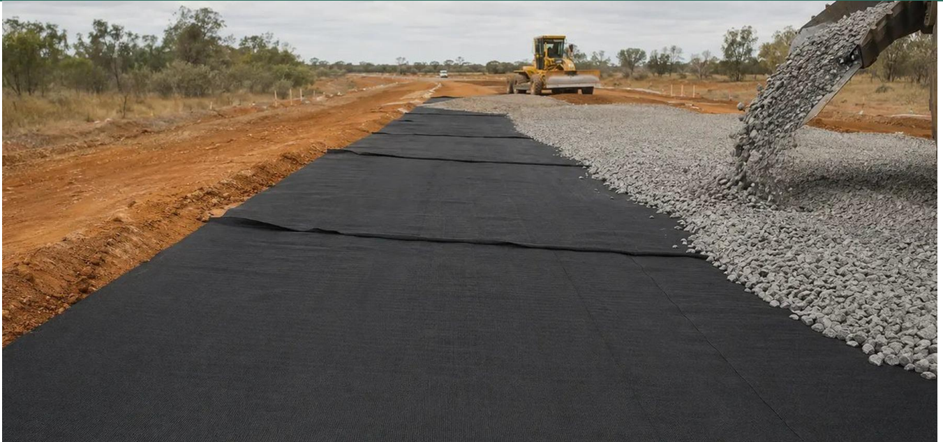
Representative woven geotextile installation beneath an unbound pavement.
