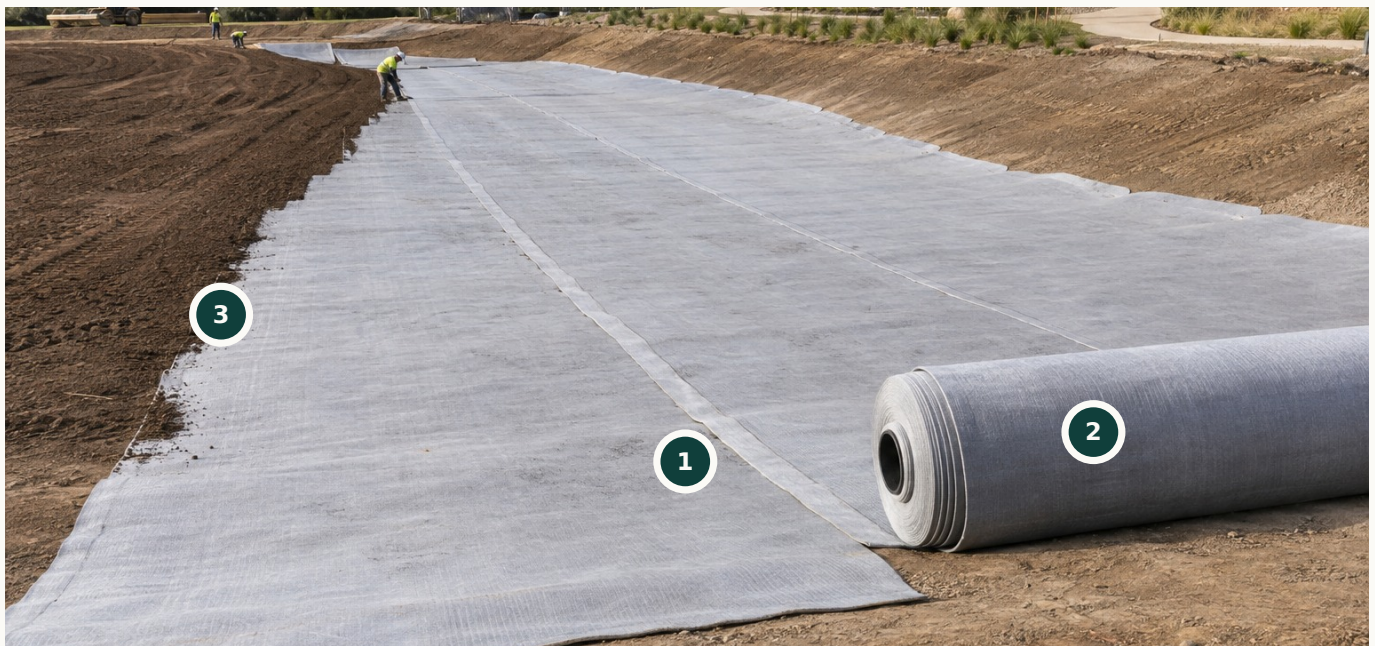
Generated installation illustration. 1 GCL layer / 2 controlled deployment / 3 progressive soil cover.
